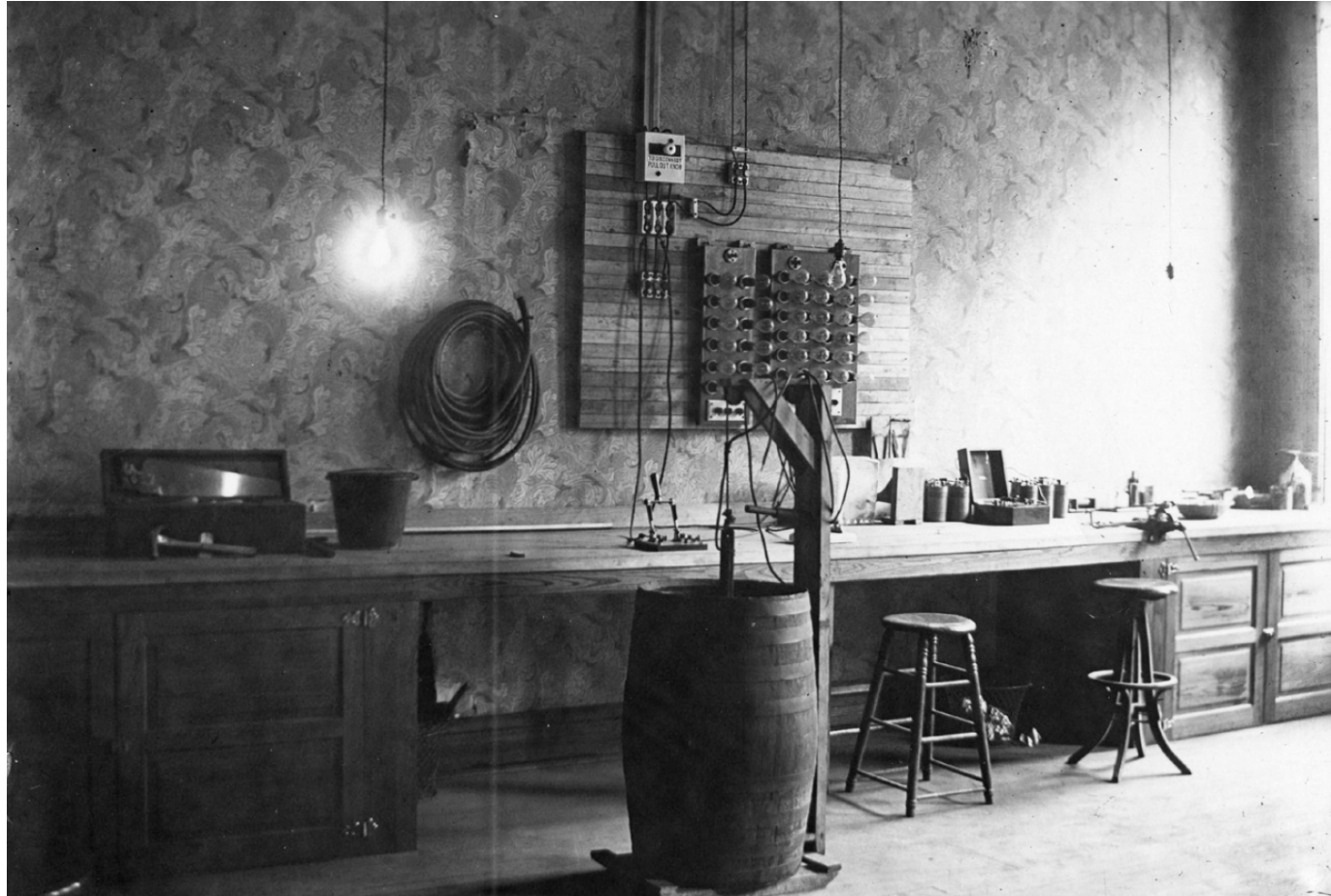
Merrill's test bench as it was when he started the Underwriters' Electrical Bureau.
